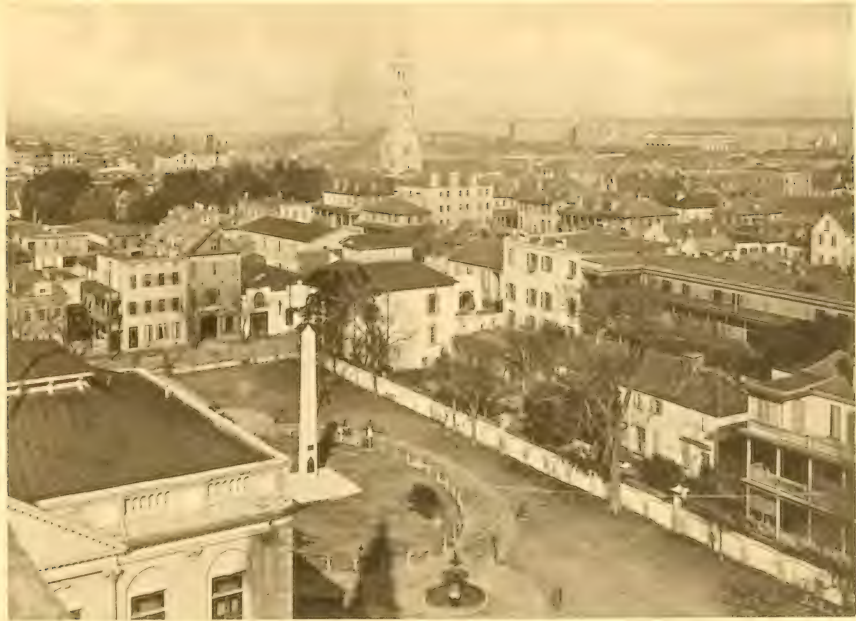
View from St. Bernard's Street.
